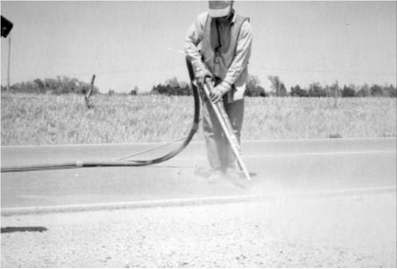
Figure 19. Sandblasting wand with wooden guide attached.
