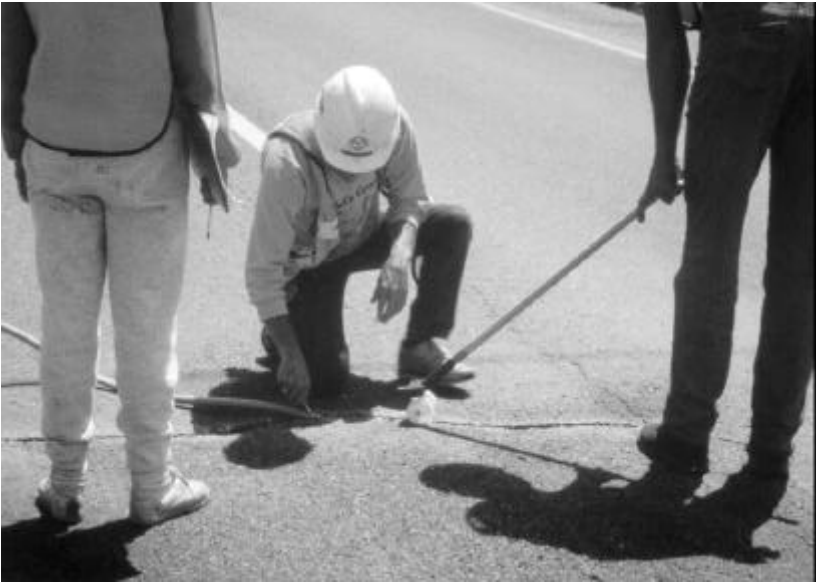
Figure 12. Backer rod installation tool.
