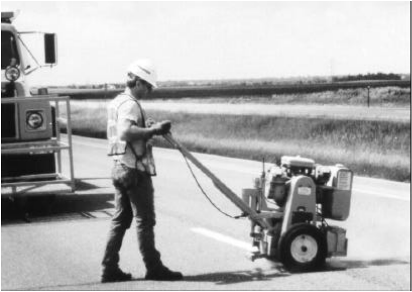
Figure 7. Rotary-impact router.
