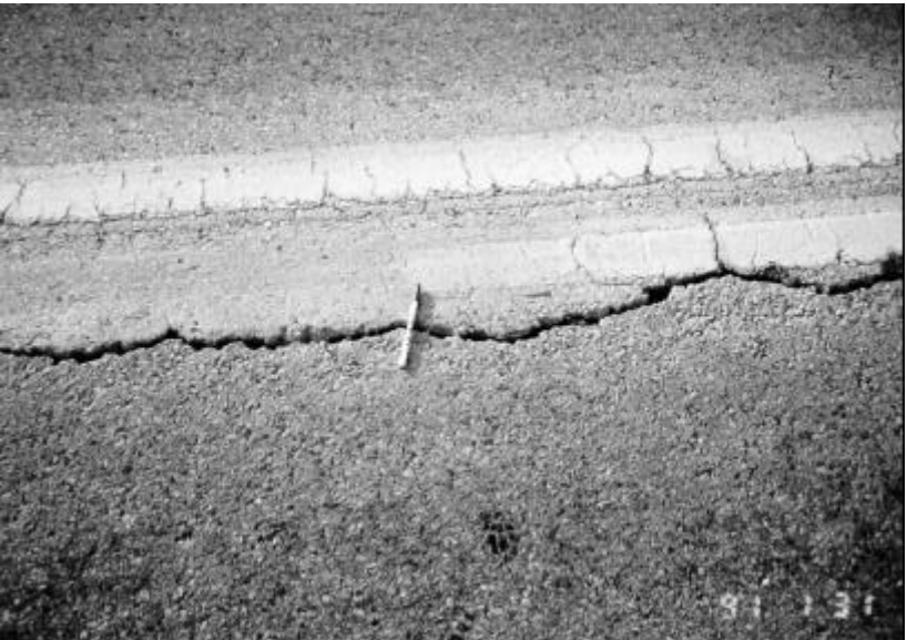
Figure 5. Pavement candidate for longitudinal crack filling.
