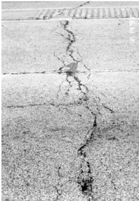
Figure 3. Pavement candidate for crack repair.
