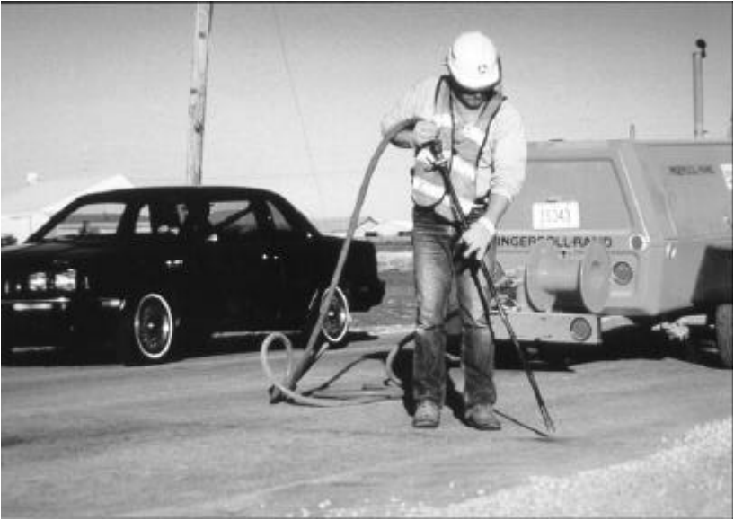
Figure 9. High-pressure airblasting using compressed air.
