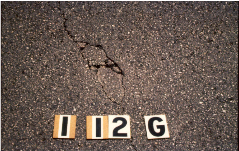
Figure 18. Primary crack accompanied by secondary crack.
