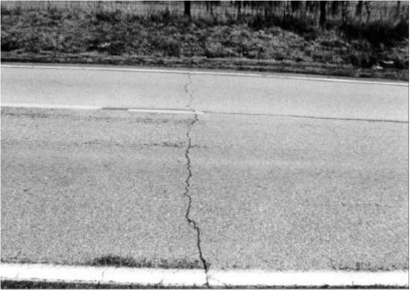
Figure 4. Pavement candidate for transverse crack sealing.
