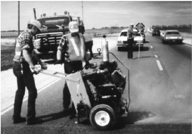
Figure 8. Diamond-blade crack saw.
