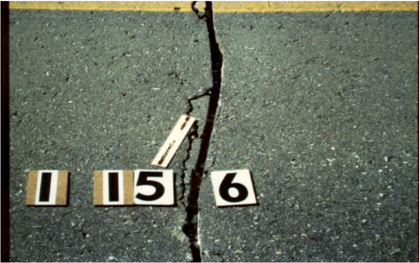
Figure 17. Crack segment missed by cutting equipment.
