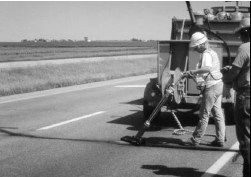
Figure 10. Hot airblasting using HCA (heat) lance.
