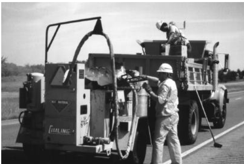
Figure 13. Asphalt kettle with pressure applicator.
