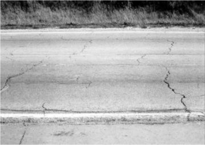
Figure 2. Pavement candidate for surface treatment: high-density cracking.
